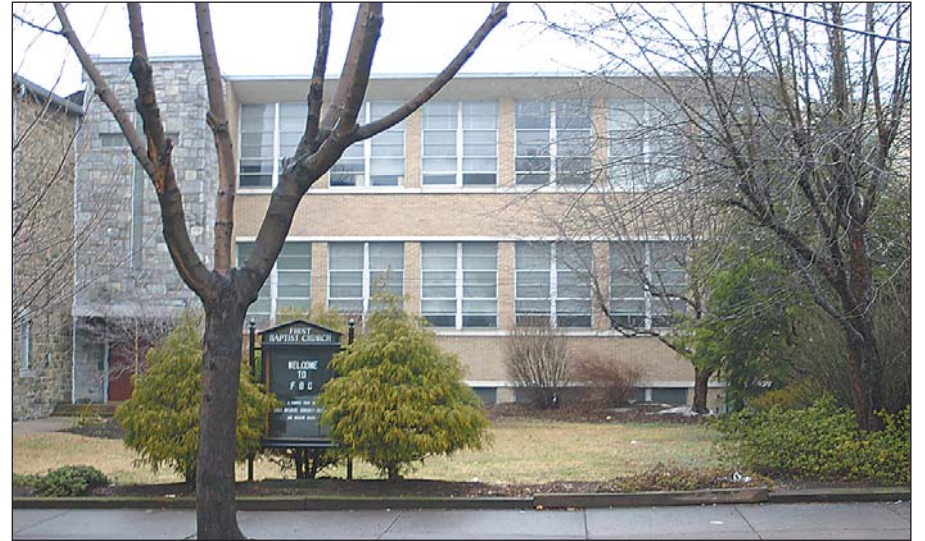
First Baptist Church at King and Charlotte streets has six spacious classrooms built in 1957 with direct access to the street and a small play area in front. The YWCA, with a gymnasium, is next door.
