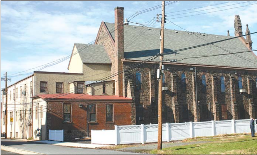
First United Methodist Church at 414 High Street has classrooms and a basement gymnasium.
